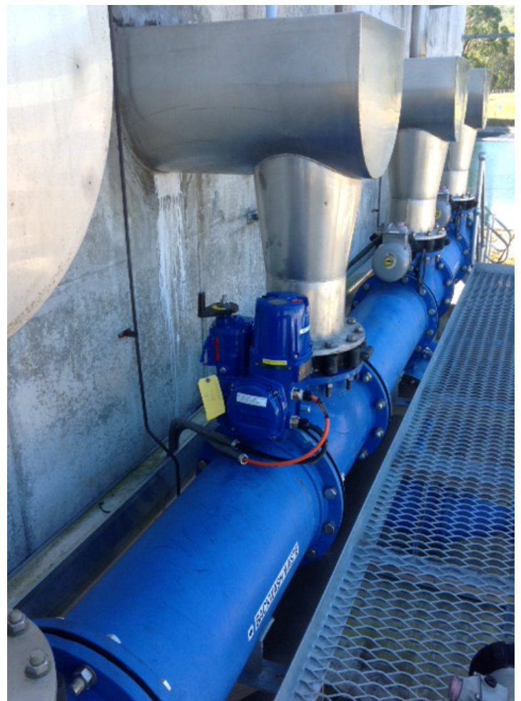
Limatorque QX on 8"600 # through conduit type gate valve
