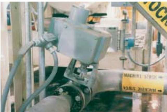
Machine chest level control valve
