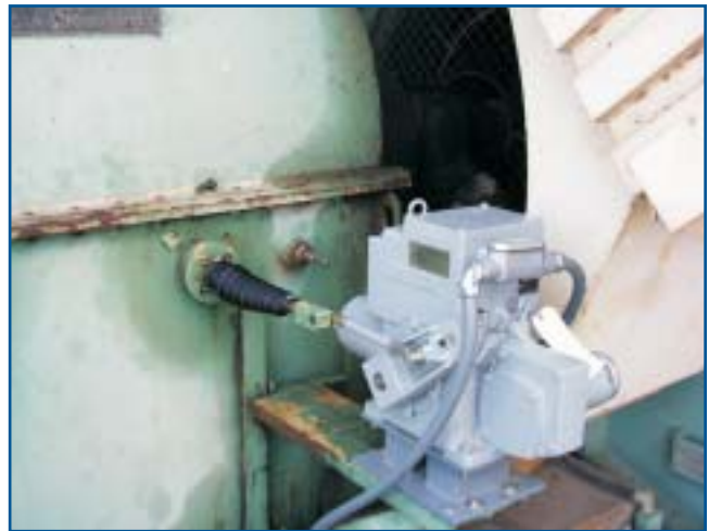
Beck drives on fluid couplings provide fast response and accurate speed control for boiler feedwater pumps and fans.
