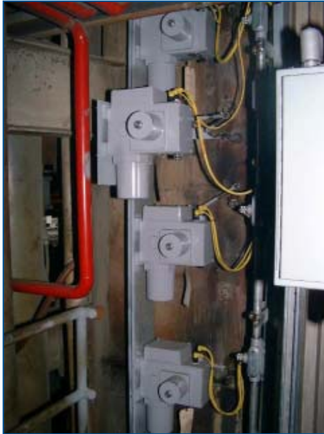
Group 11 drives provide precise control of secondary airflow on windbox dampers.
