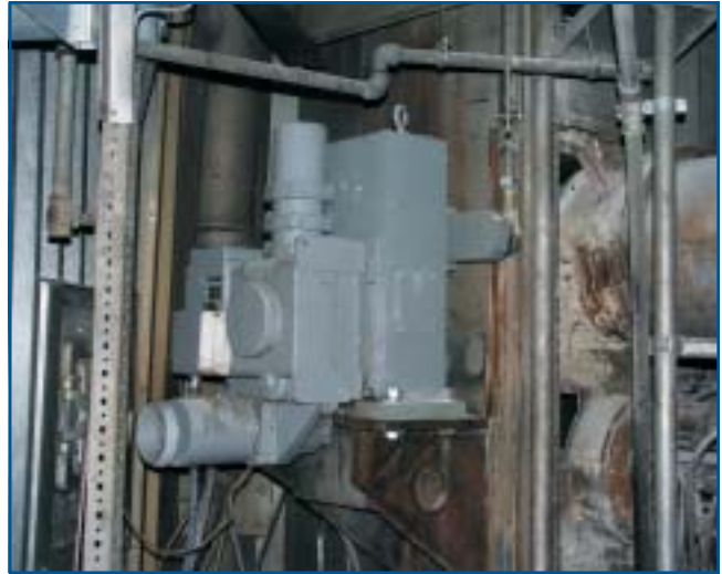
Group 11 drives deliver stable control for burner tilts.
