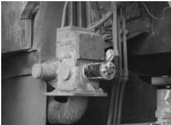
Beck drive with CPS cover removed
